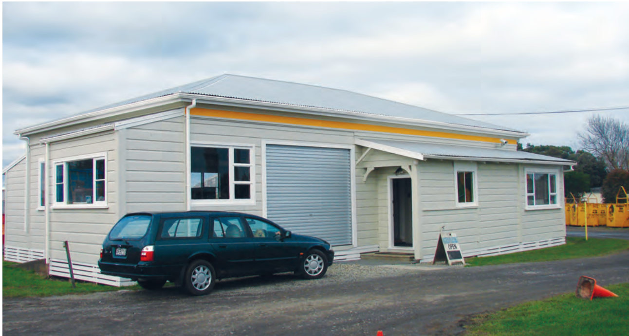
Ingram Contracting's premises have been renovated for the 50th anniversary, with many thanks to DR (Jack) Gray, Hawera for their expert painting.
