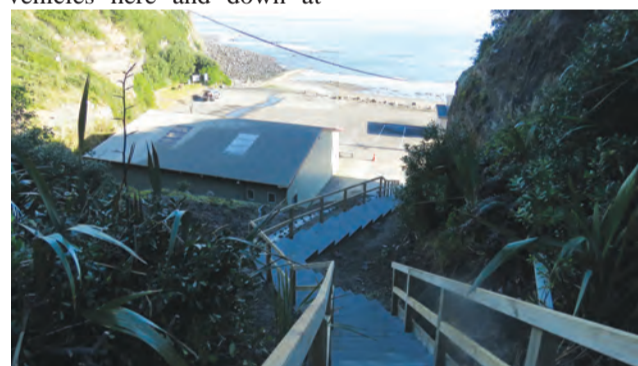
Middleton Bay. The public toilets are at left.
